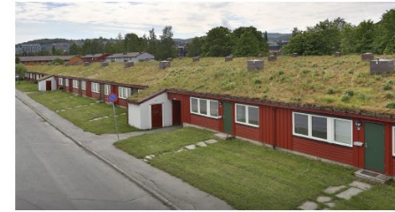
(b) Green roof at Frode Rinnans veg Student Village (Photo: SIT.no)
